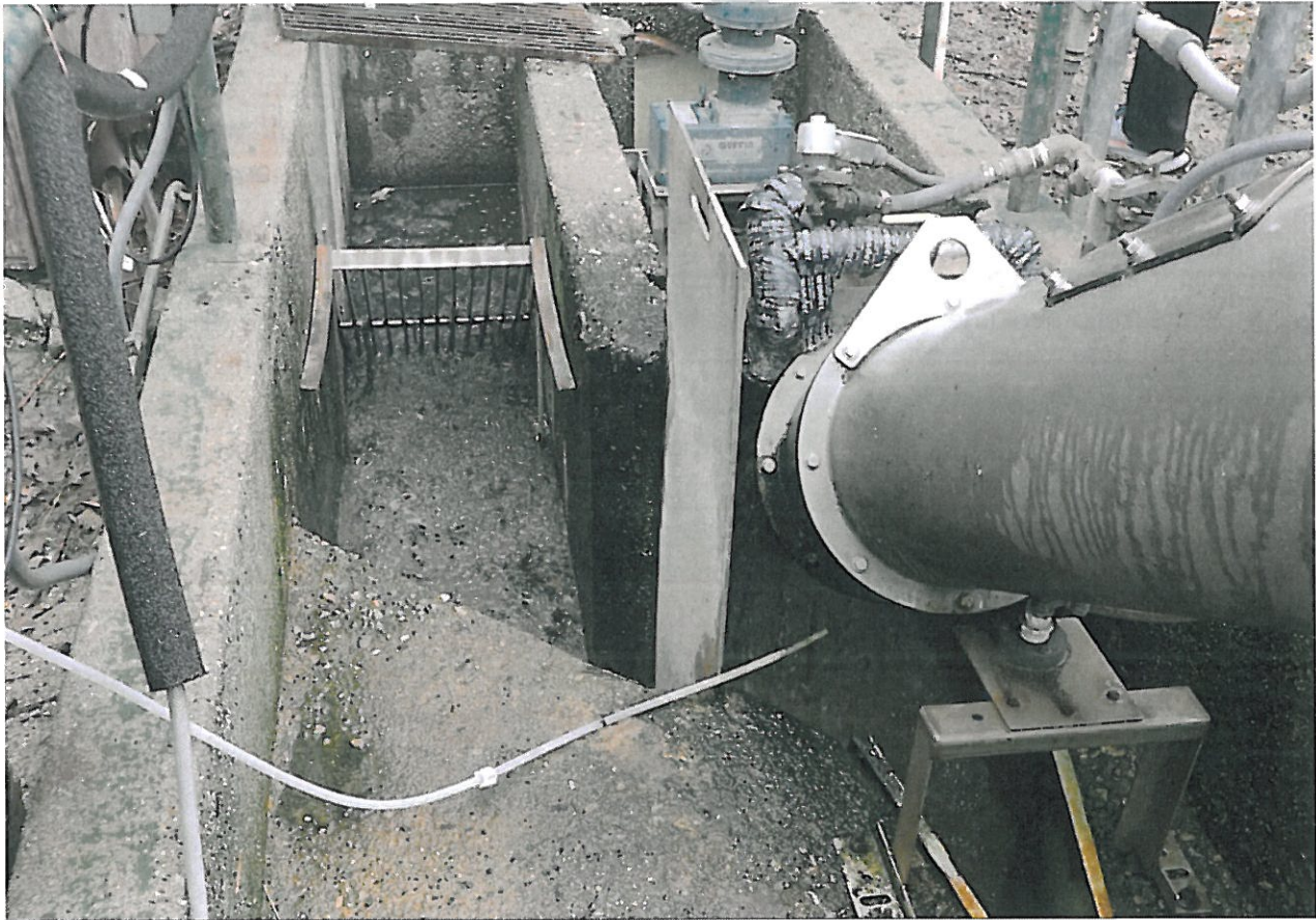
Figure 3: Existing Headworks Bypass Channel And Bar Screen
