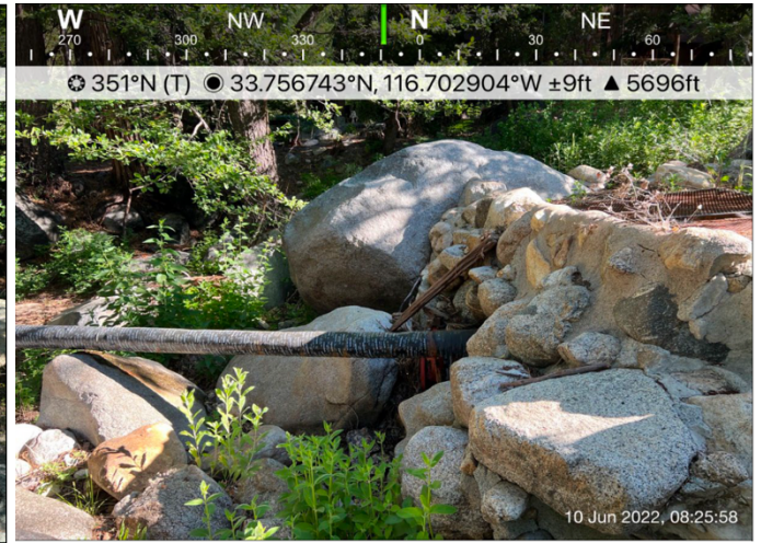
Photo 4. View of the water diversion structure and existing pipeline.
