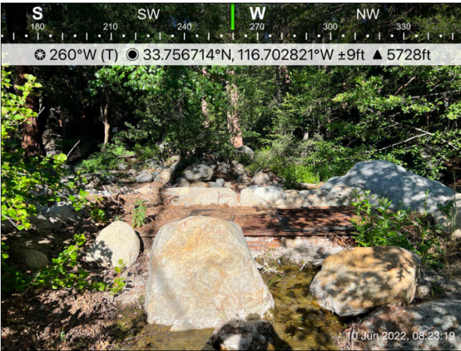
Photo 3. View of the water diversion structure.
