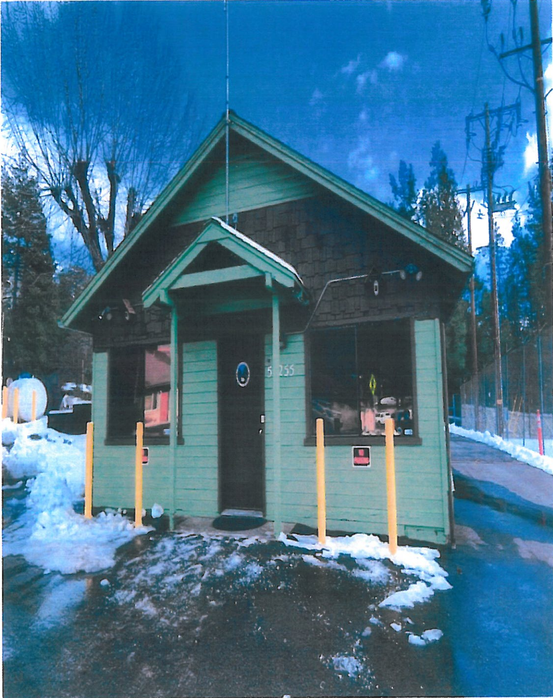
The property to be inspected/tested
