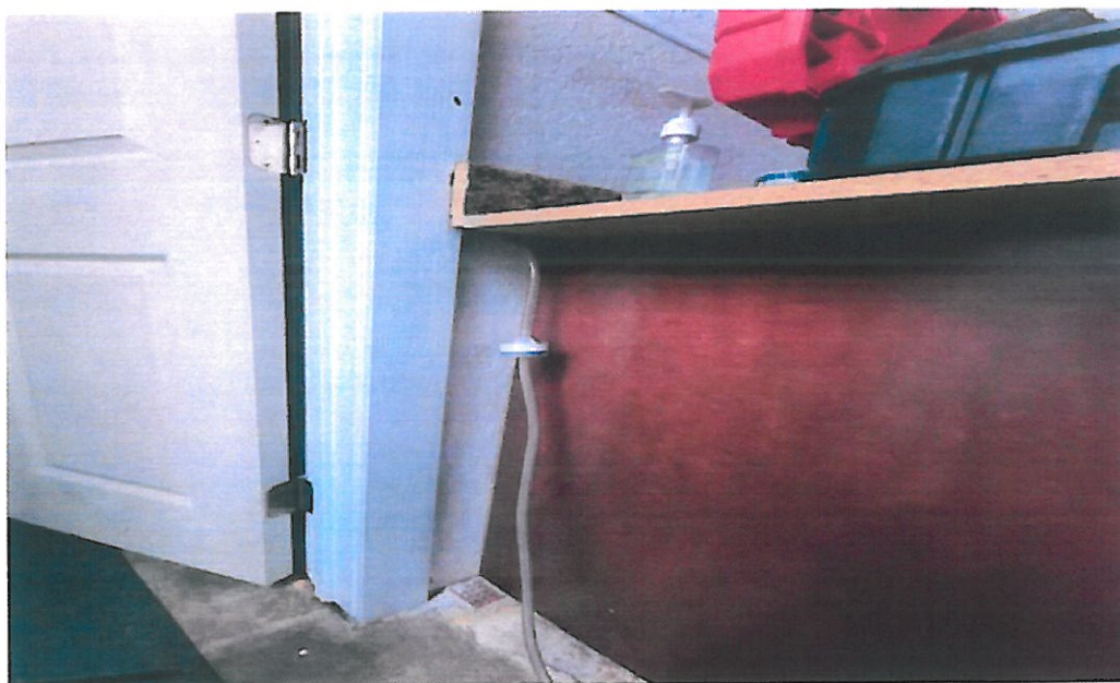
The inside air sample was taken at the hallway wall cavity
